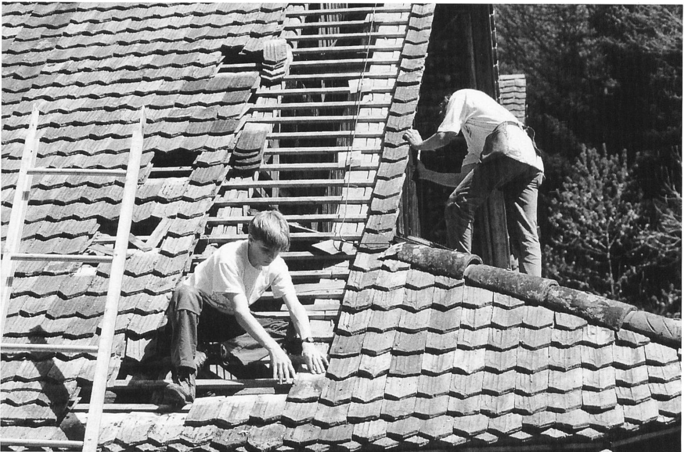
Dachrenovation Ziegelhütte Meienberg, Cham (Phototec Pfeiffer, Steinhausen).
